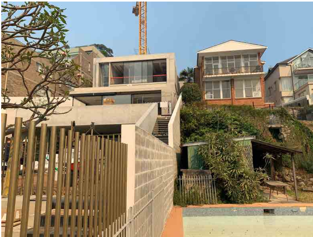
View west of the interface with 3 Bay View Street.
