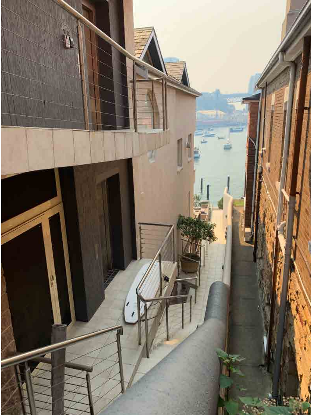
View east from the street frontage towards 7 Bay View Street interface showing the excavated lower level below the ground level of the subject site.
