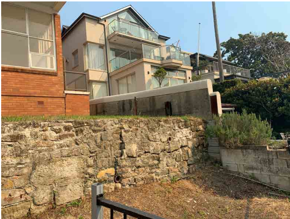
View north-west towards 7 Bay View Street interface.
