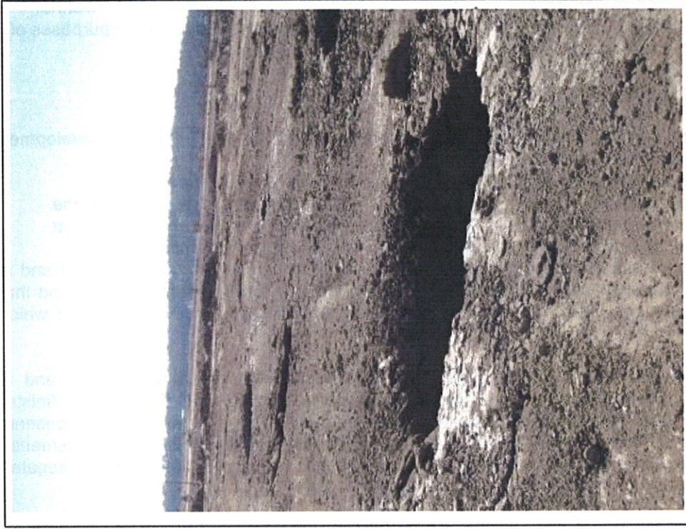
Figure 4 – Ground Treated by Dynamic Compaction
