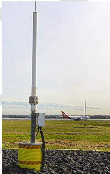
Figure 30: GBAS Ground Infrastructure
