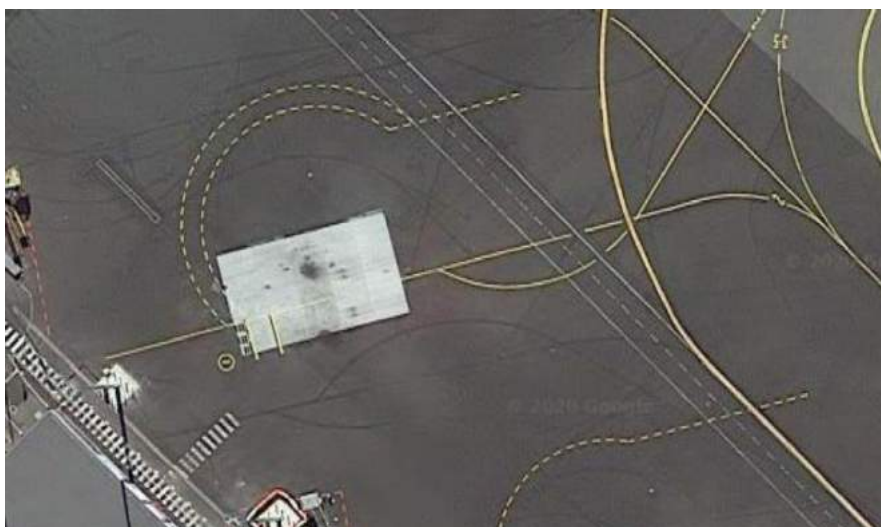
Figure 24: Code C Concrete Panel Extent (Hobart Airport, Google)
