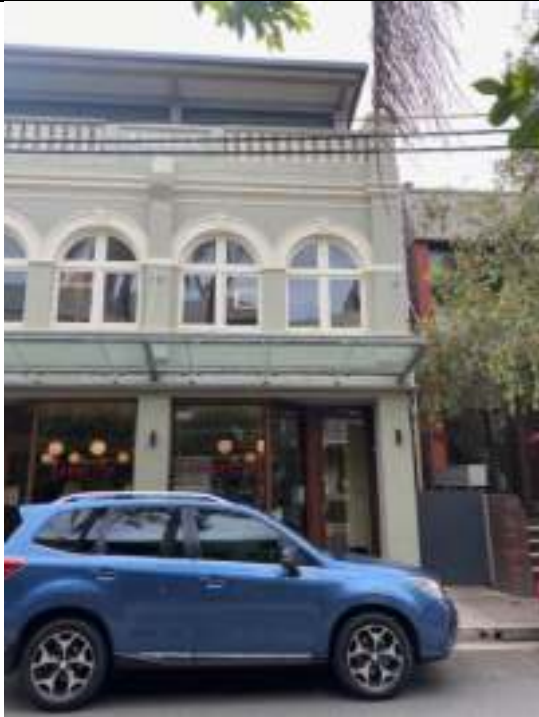
Photo 3: Existing northern entrance and side service entrance
