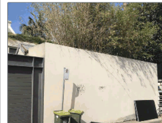
No. 30 GLENVIEW LANE RETAINING WALL
