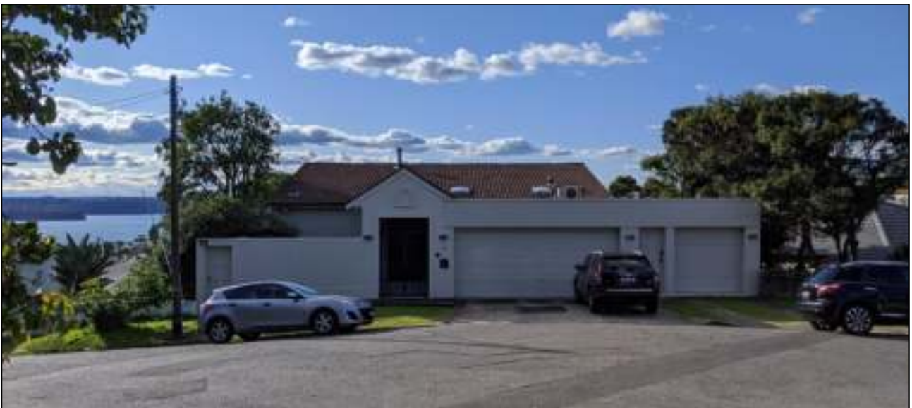
Figure 2: View of subject site from Olphert Avenue
