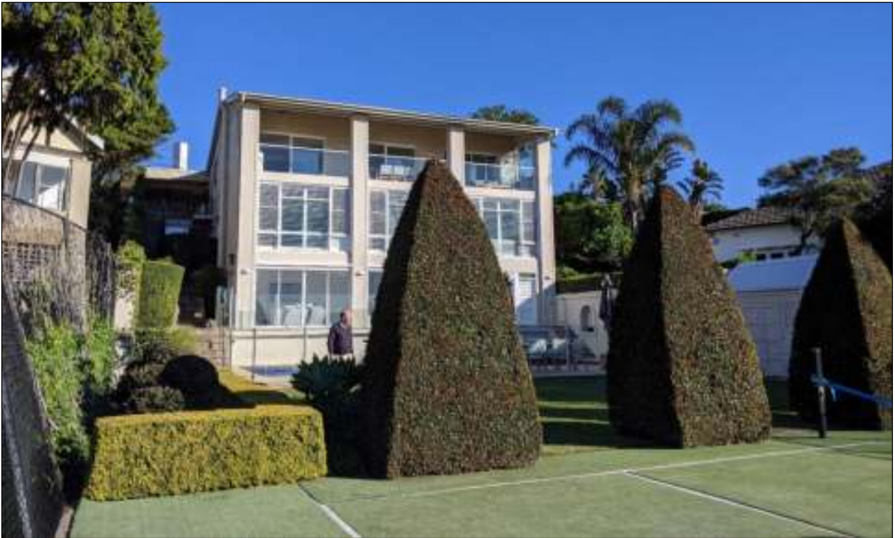
Figure 3: Rear elevation of the existing dwelling
