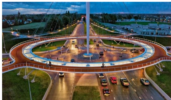
The 'Hovenring' in Eindhoven, The Netherlands, is an elevated roundabout for cyclists so they can safely cross the busy road intersection.
