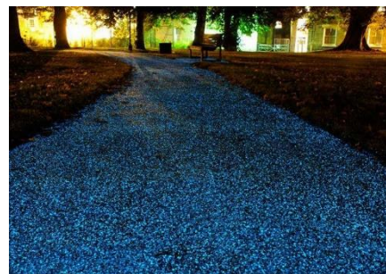
Spray-on 'Starpath' glow-in-the-dark product being trialled in Cambridge, UK in 2013.
