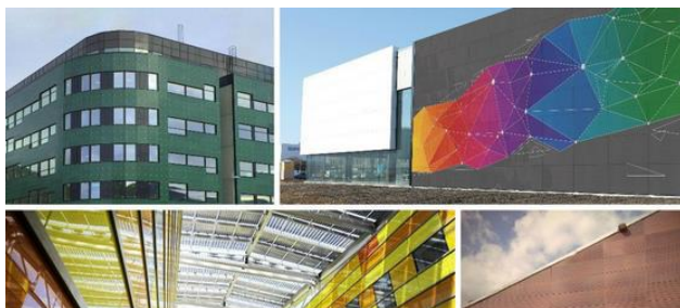
Swiss company, Solaxess, produces coloured and white-finish nanotechnology films to fit to traditional solar panels which alter their appearance without inhibiting function.
