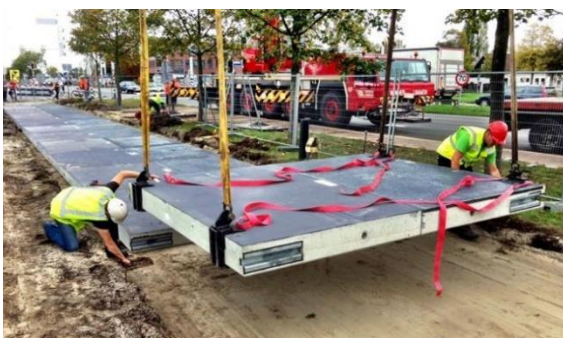
'Solaroad', the world's first solar panel bike path installed in 2014 in Amsterdam, The Netherlands.
