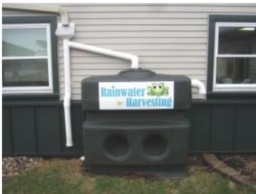
Examples of residential and commercial rainwater harvesting systems for toilets, fire sprinklers etc.
