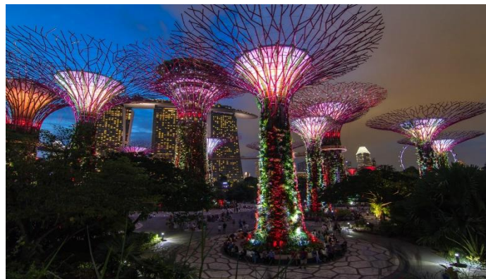
'Supertree Grove' at Gardens by the Bay, Singapore. These structures combine technology, nature, and functionality. The trunks are covered with vertical gardens, incorporated solar panels store energy to light the Gardens at night, their canopies provide shade during the day, and they collect rainwater for use in irrigation in the Gardens.
