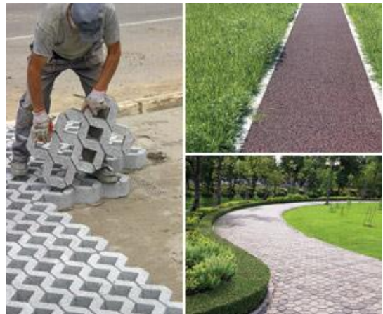
Examples of permeable paving applied in private and public driveways, footpaths and open spaces.
