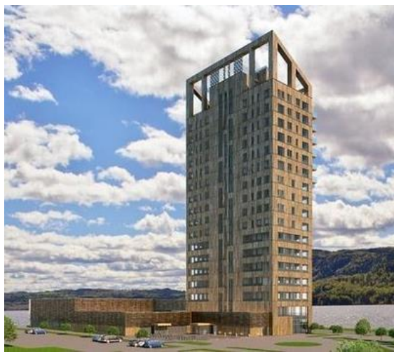
Mjøsa Tower, is a mixed-used, 18-story building in Norway. Opened in 2019, it is the World's tallest mass timber building.
