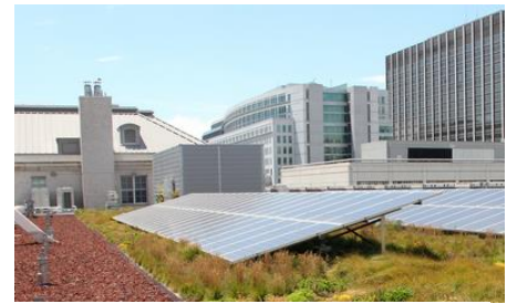
Solar combined with green roof on top of the US Federal Building in San Francisco
