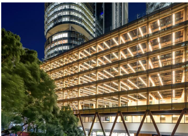
The first and largest commercial mass timber building in Australia is International House in Sydney.
