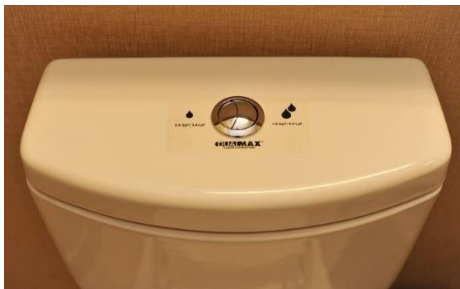
Standard toilet installs in Australia now include dual flush options to help save up to 70% of water use
