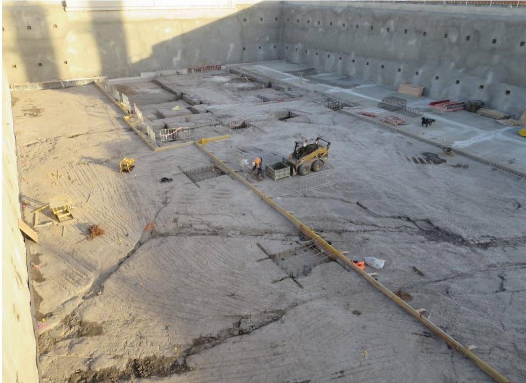
Photo 5: Excavated floor in fresh Ashfiled Shale with typical geological structures
