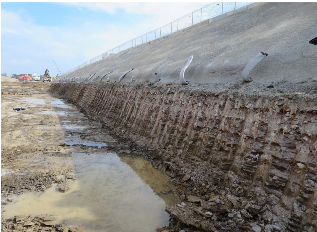
Photo 2: Excavation face in weathered Ashfield Shale
