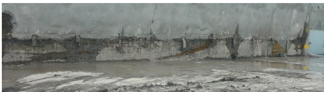
Photo 4: Excavation face in fresh Ashfield Shale with jointing
