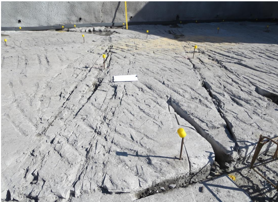
Photo 6: Excavated floor in fresh Ashfiled Shale with typical geological structures
