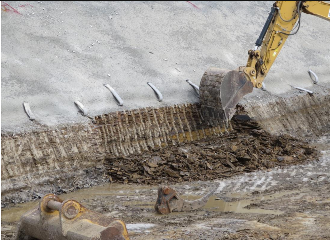
Photo 1: Excavation face in weathered Ashfield Shale
