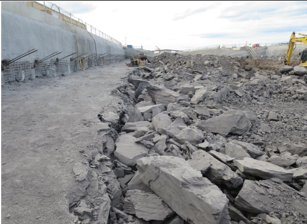
Photo 3: Bulk excavation of fresh Ashfield Shale
