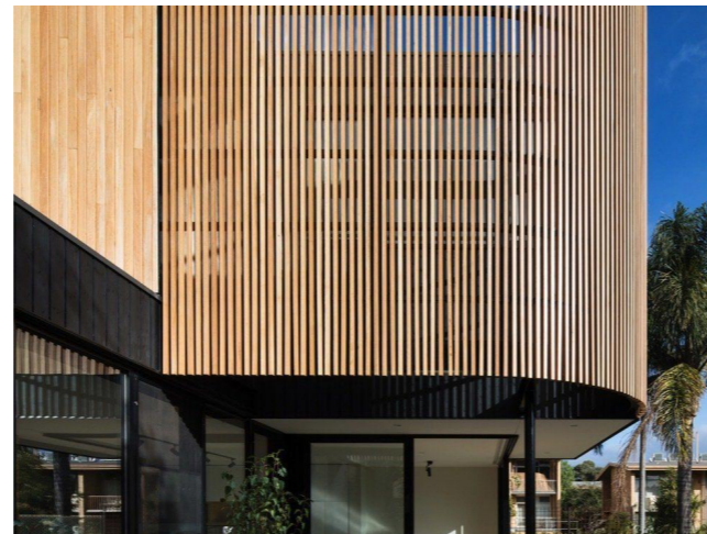
TB1 TIMBER BATTEN SCREEN
