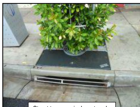
Street tree passively watered from stormwater runoff
