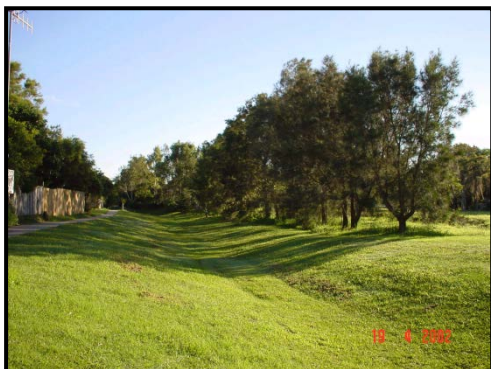
Figure B9.8 – Example of drainage line that encourages the use of natural materials.
