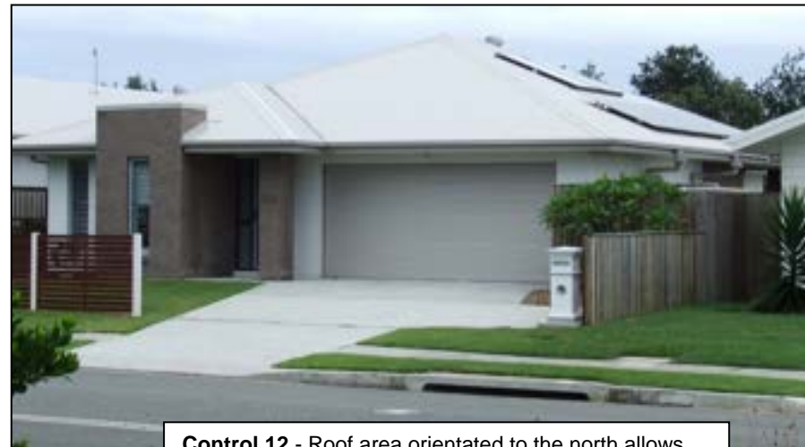
Control 12 - Roof area orientated to the north allows for both solar hot water system and photovoltaic cells.
