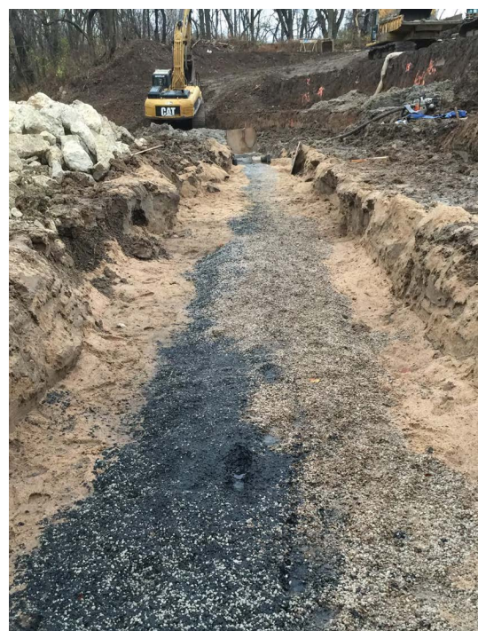
Groundwater Remediation (Permeable Reactive Barrier)
