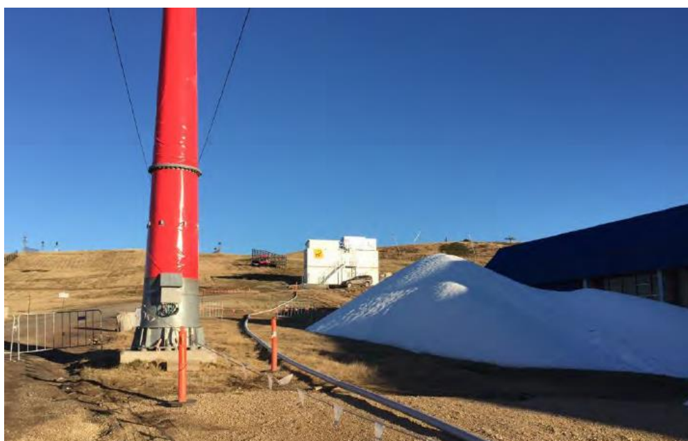
Figure 5 | Example of stockpile and pipes connected to Snowfactory (Source: Applicant's documentation)
