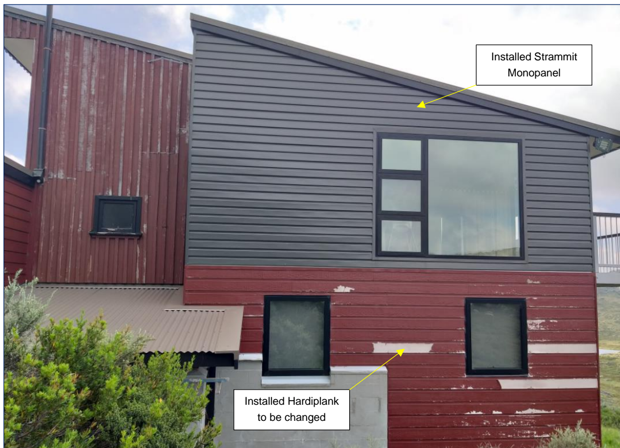
Figure 6 | Existing southern elevation illustrating part of works completed and area to be replaced with Stramit Monopanel (Source: Department inspection - 2020)
