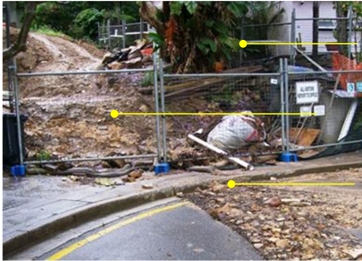
Inadequate erosion and sediment control measures
