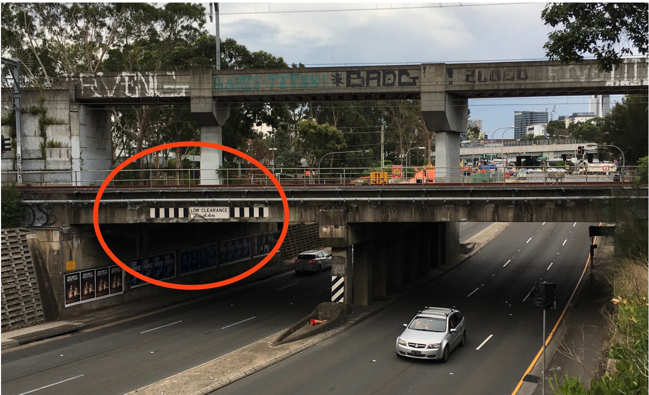
Photo 1.1 showing clearance sign and damage to sign by collisions. Taken by residents.
