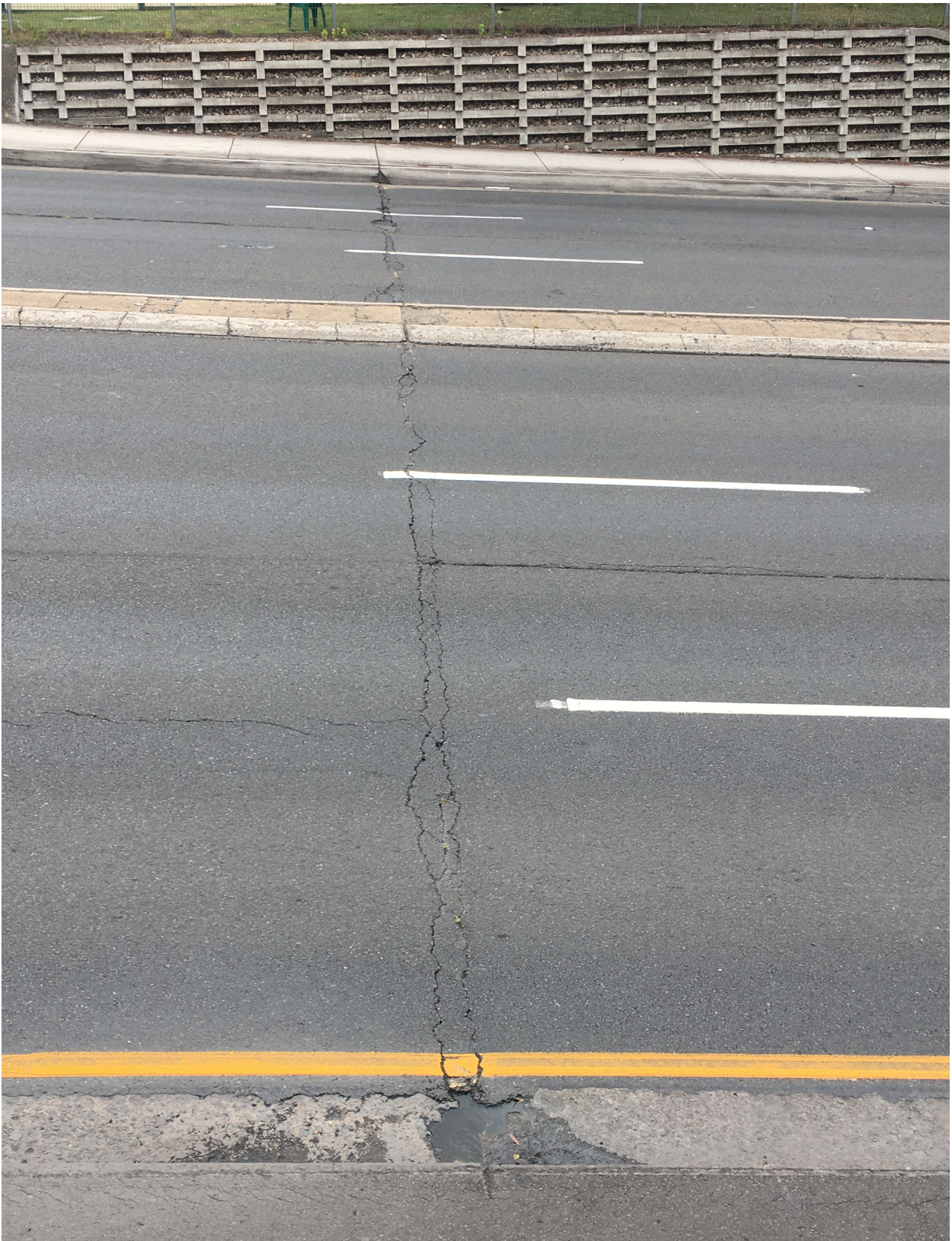
Photo 2.1 showing crack and potholes. Taken by residents.
