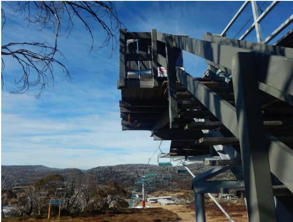
Figure 7 – View of the lift hut to be relocated and platform to be cut back
