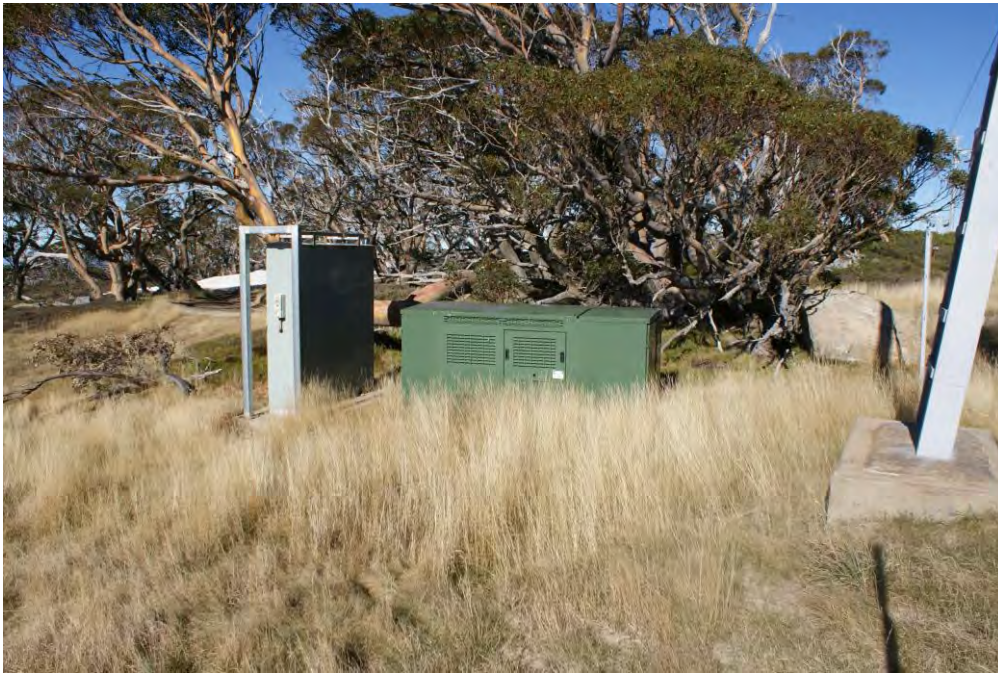
Figure 15: Example of an electrical transformer
