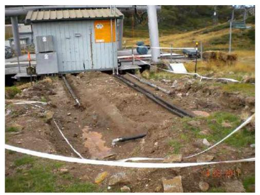
Figure 34: Underground fuel tanks to be removed
