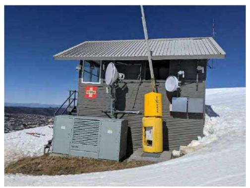
Figure 39: Electrical transformer to be replaced and upgraded
