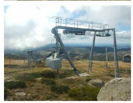
Figure 9: Eyre T-bar top station bullwheel to be relocated down the slope
