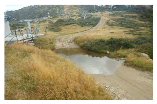
Photo 1: The crossing of Perisher Creek will be upgraded to improve construction access and reduce water quality impacts that would otherwise be associated with construction access. The upgrade will be similar to existing crossings further downstream i.e. near the Quad Express Chairlift.
