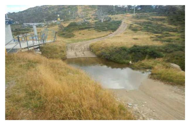
Photo 5: The crossing of Perisher Creek will be upgraded to improve construction access and reduce water quality impacts that would otherwise be associated with construction access. The upgrade will be similar to existing crossings further downstream (i.e. near the Quad Express Chairlift).
