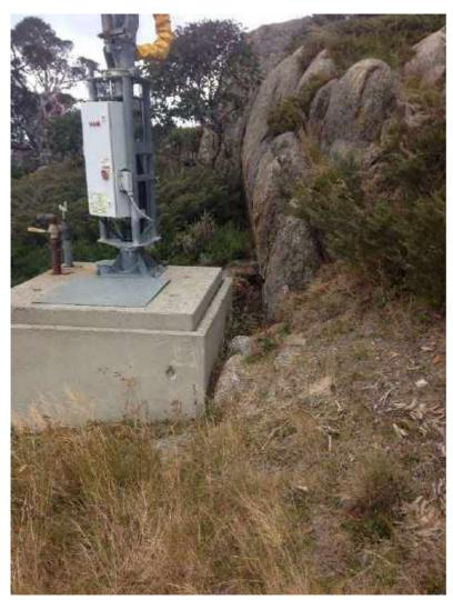
Plate 10 (Pylon #6, snow lance base downhill of proposed location showing construction against granite outcrop.)
