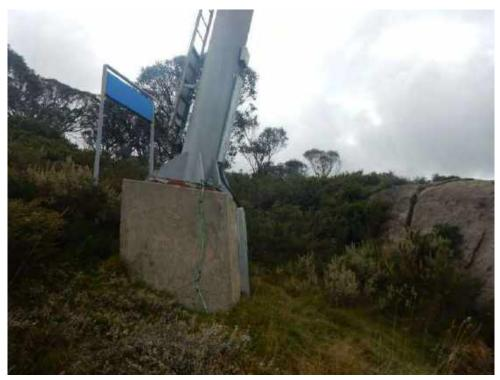
Figure 33: Example of concrete footings to be removed
