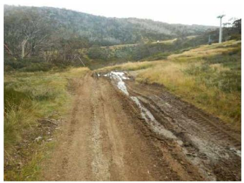
Figure 46: Existing access road requires upgrading for construction and operation of the new lift
