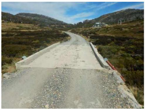
Figure 47: Culvert constructed downstream for access to the Leichhardt Chairlift
