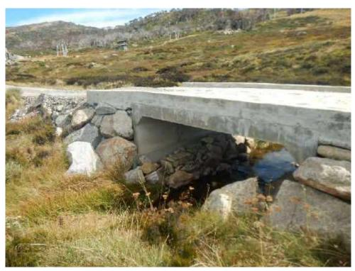
Figure 48: Culvert constructed downstream for access to the Leichhardt Chairlift
