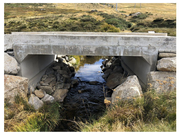
Similar culvert 800m downstream
