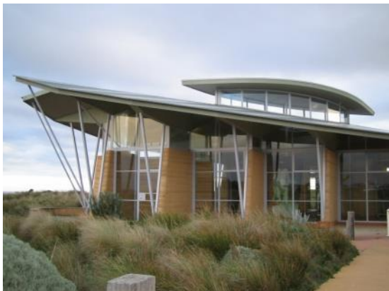
Openable roof top windows improve natural ventilation
