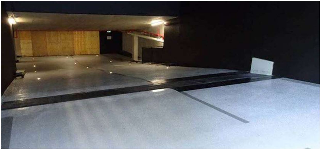
This 500mm high FloodBreak Slimline was installed in Brisbane, car park entry new high rise apartment building, downwards slope.
