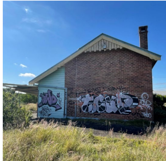
Photograph 4-15 West elevation of early 1869 brick school building showing gabled roof with simple gable roof end decoration and timber lean-to
