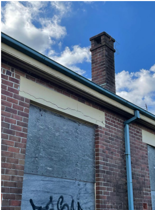
Photograph 4-16 closer view of south elevation brick detailing and chimney, timber window frames removed and boarded up
