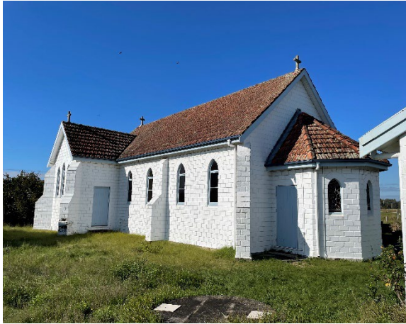
Photograph 4-1 North elevation of St Saviour's, brick face, steep gabled roof and lancet arch windows, circular apse
