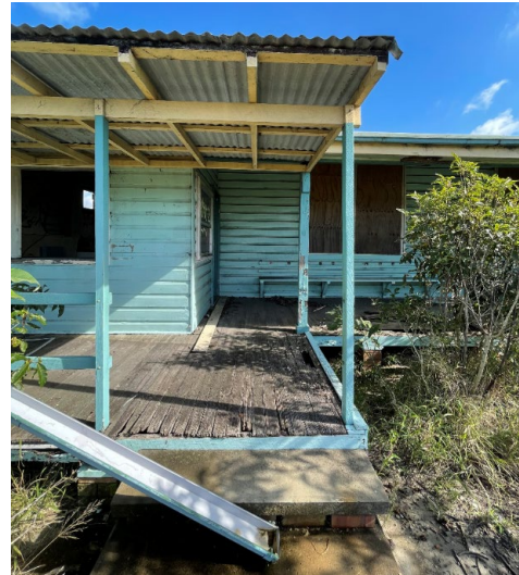
Photograph 4-19 horizontal timber cladding and timber post verandah clad in corrugated iron
