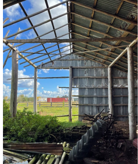
Photograph 4-11 Internal view of barn showing timber framing
