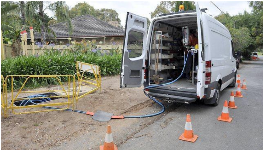
Figure 5-6 | Splicing Van Accessing a roadside pit
