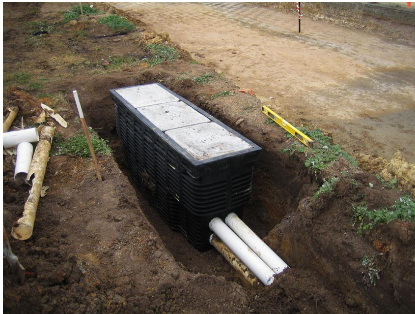
Figure 5-5| "9 Pit" with multiple P100 conduits being installed
