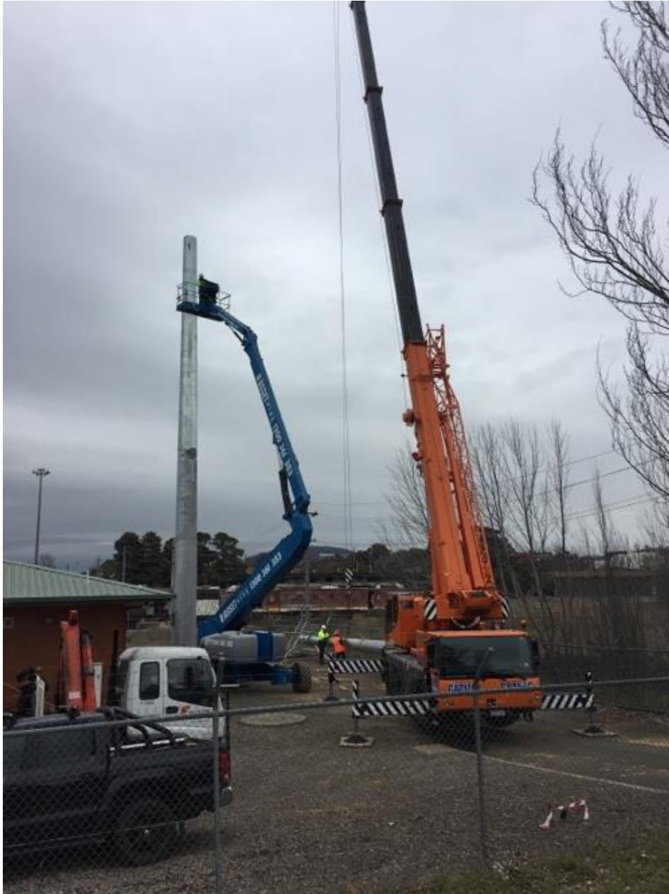
Figure 5-3 | A crane and an EWP assembling a mobile tower
