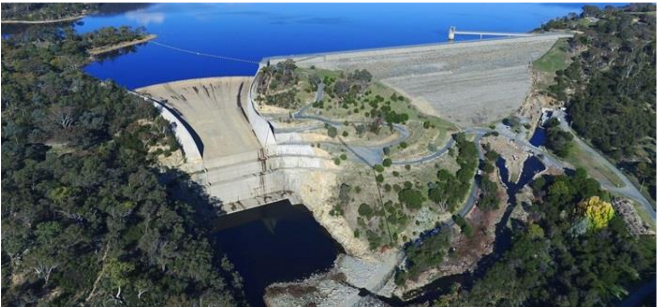
Figure 6-1 | Googong Dam Spillway (source: Icon Water 2022)
