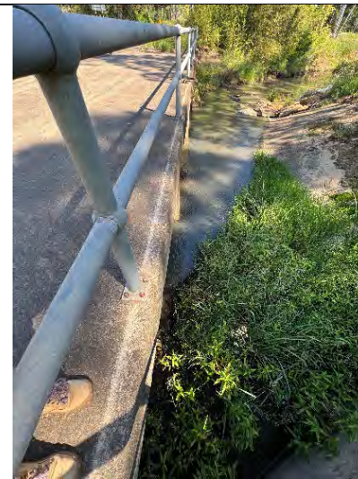
Photograph 06. Grange Avenue (Bells Creek Crossing) looking downstream
