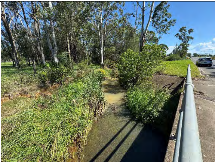
Photograph 05. Grange Avenue (Bells Creek Crossing) looking upstream
