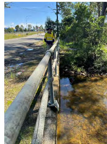
Photograph 02. Townson Road (Bells Creek Crossing) looking downstream.
