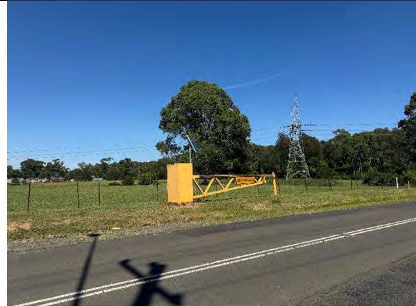
Photograph 10. Grange Avenue Flood Gate (Eastern Creek Crossing)
