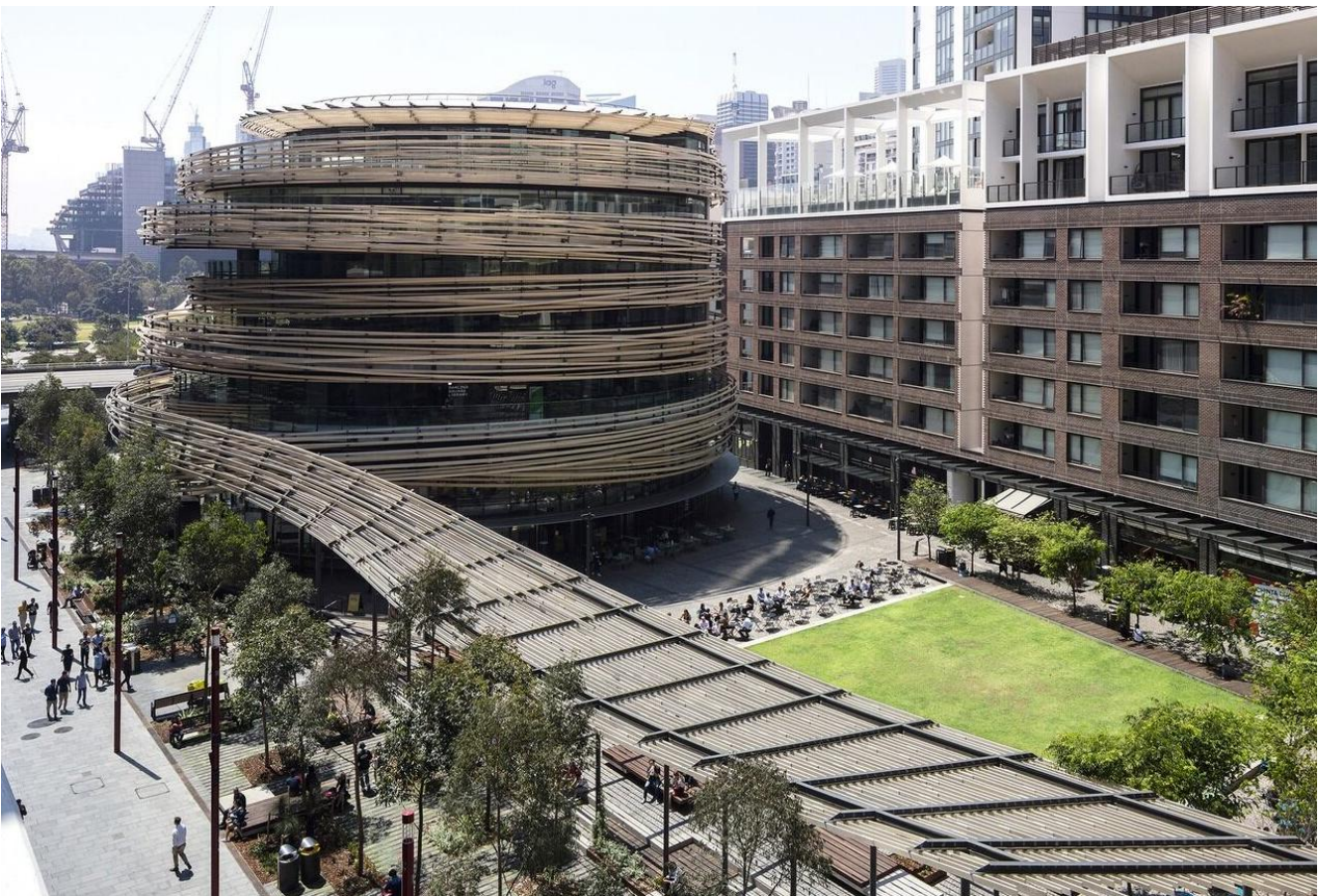
Figure 23 The Exchange Darling Square by Kengo Kuma & Associates & Aspect Studio
