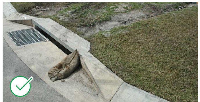
A good example of gutter protection using a sandbag. Source: Catchments and Creeks Pty Ltd.
