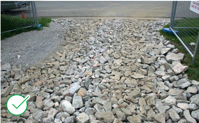
A good example of a stabilised site entry/exit point. Source: Catchments and Creeks Pty Ltd.
