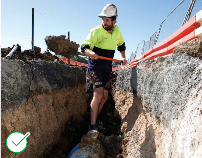
A good example of a construction worker installing a service trench.
