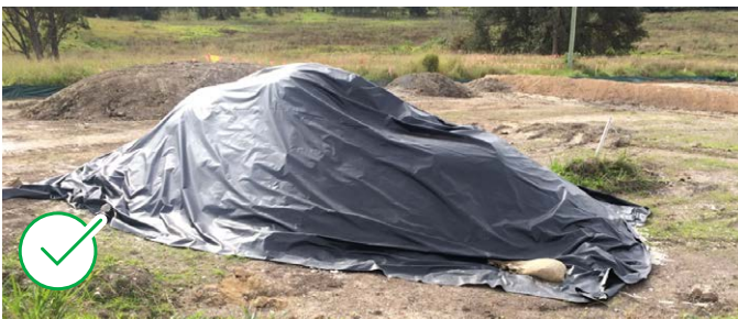
A good example of stockpile management, where a sediment stockpile has been securely covered and a bund installed downhill. Source: Department of Primary Industries and Regional Development – Fisheries.
