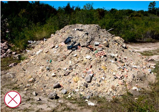
A poor example of stockpile management, where a sediment stockpile is left exposed.
