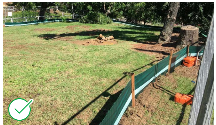
A good example of a sediment fence that has been appropriately installed.
